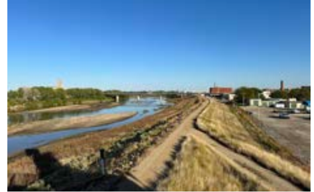
Cut and laid stone to protect the levee
